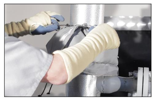
3. PULL OUT A SUFFICIENT AMOUNT OF SS WIRE AND TWIST THE END OF IT INTO A LOOP. TRIM THE SS WIRE AT THE BASE OF THE CYLINDER AND ATTACH IT TO AN SS LACING HOOK ON THE ISOCOVERS INSULATION JACKET:
