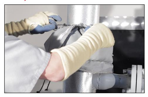
3. PULL OUT A SUFFICIENT AMOUNT OF SS WIRE AND TWIST THE END OF IT INTO A LOOP. TRIM THE SS WIRE AT THE BASE OF THE CYLINDER AND ATTACH IT TO AN SS LACING HOOK ON THE ISOCOVERS INSULATION JACKET:
